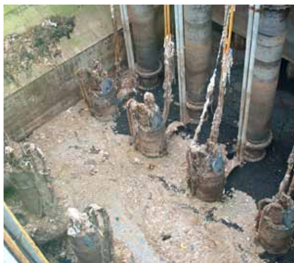
Pump station with accumulation of floating debris.
